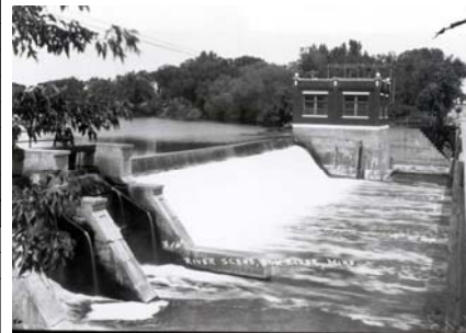
The Elk River Falls Hydropower Plant (1920)
