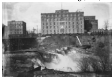
Falls utilized but eroding (1902)
