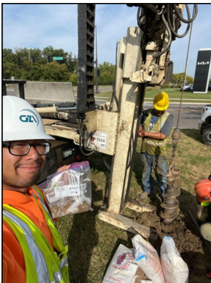
Monitoring well installation field work in Brooklyn Park, MN, with Bergerson-Caswell drillers Greg and Dave
