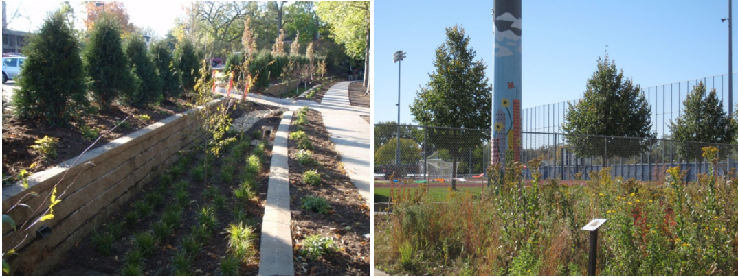
Photo of Janet Wallace Fine Arts Parking Lot stormwater project and Olin Rice prairie.
